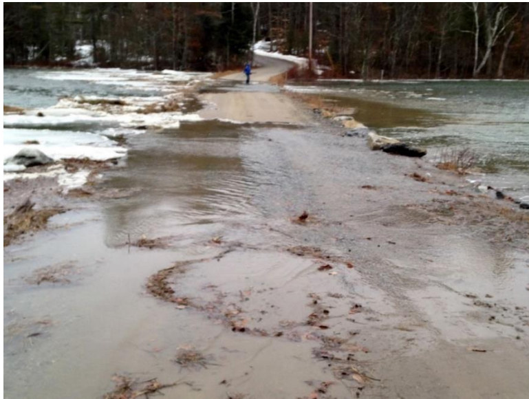
Long Reach Lane
