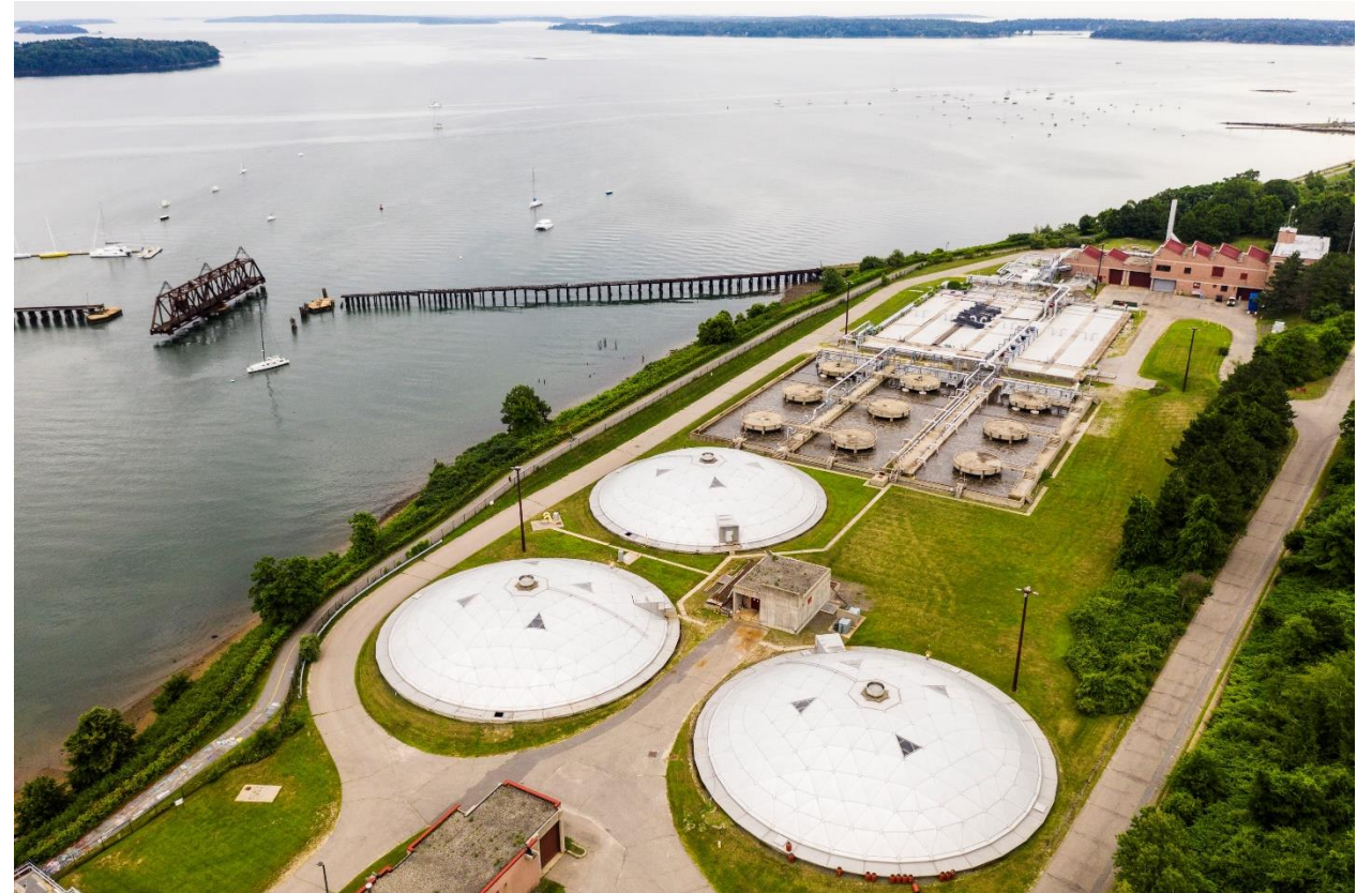
East End WWTF, Portland, ME
